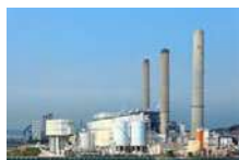
Thermal Power Plants
