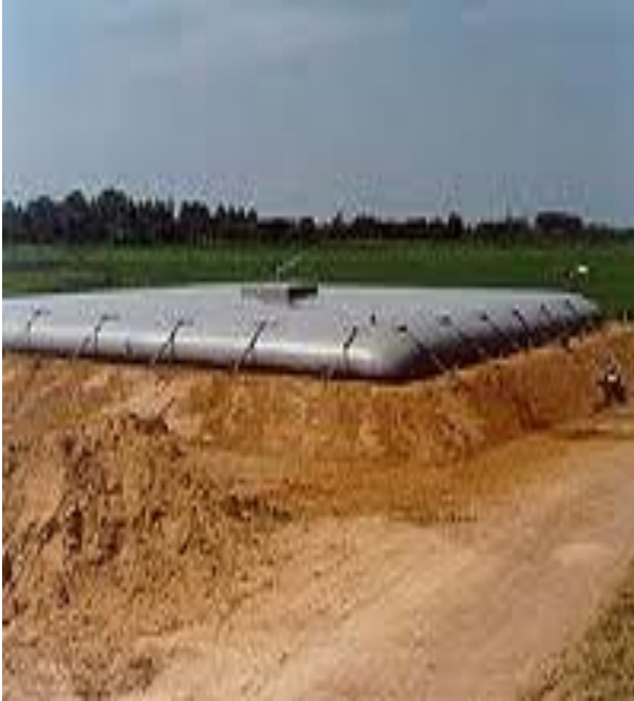
Bag storage tank
