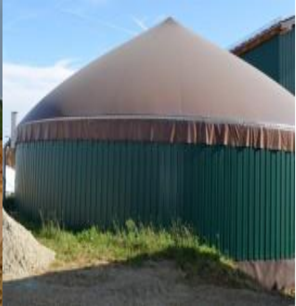
Digestate storage tank with tent cover
