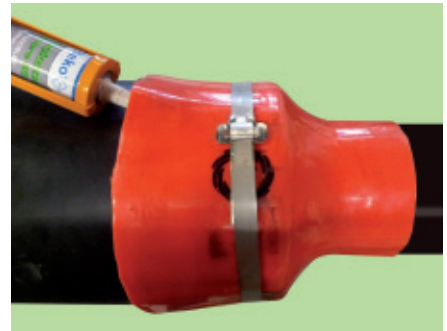
3. Inject sealing adhesive under the sleeve all around
