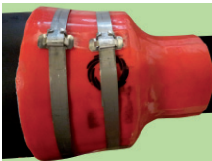
4. Fix second strap on the casing pipe (smoothen sealing adhesive on the edges)
