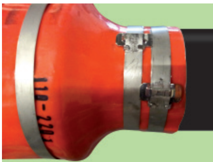
7. Fix the second strap on the carrier pipe at the end
