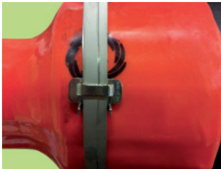
2. Put straps around the seal and push into the closure
