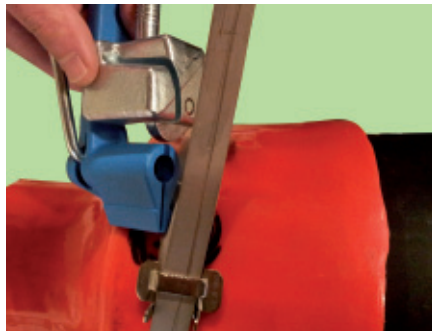
3. Treat strap tightly and pitch sideways into the tension pincers. Then push the pincers up to the closure.
