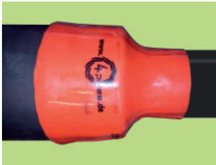
1. Push sealing sleeve over carrier and casing pipe
