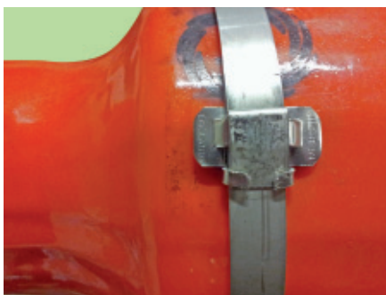
8. Revert security clips to fix the tape
