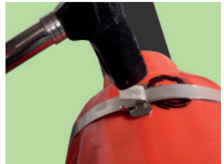
7. Revert tape with a hammer into the closure clip.
