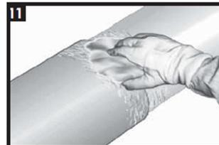
Clean the roughened surface to remove any polyethylene or sand particles, using a dry grease and lint-free rag.
