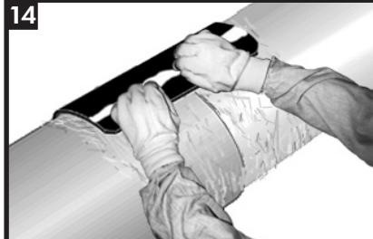
Centre the sleeve over the area to be sealed (casing pipe/PE pipe) and press the underlap into place. Remove the remaining release liner from the sleeve.
