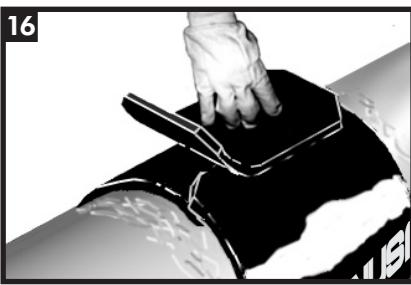
Gently heat the closure and pat it down with a gloved hand. Repeating this procedure, move from one side to the other. Smooth any wrinkles by gently working them outward from the centre of the closure with a roller.
