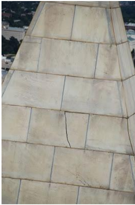
A one-inch wide, four-foot long crack was spotted Wednesday in the Washington Monument's pyramid, near the very top of the 555-foot obelisk. (U.S. Park Police Aviation)
