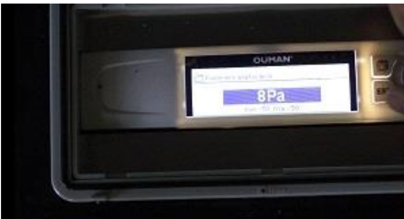
Picture 3. The pressure difference can be set with 1 Pa accuracy using the display of the control unit
