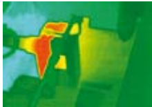
Motor: Bearing Problem
