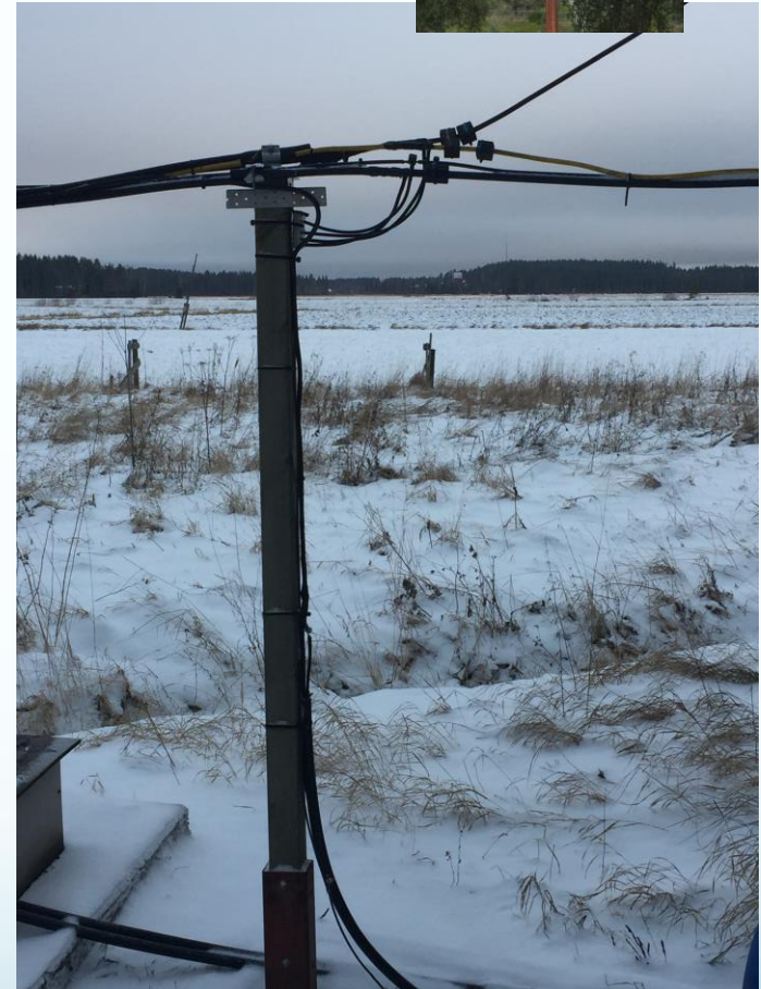
Cables grounded at mast base.
