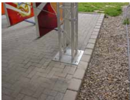
Anchoring to the ground with impact dowels
