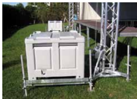
Ballasting with water tanks and booms
