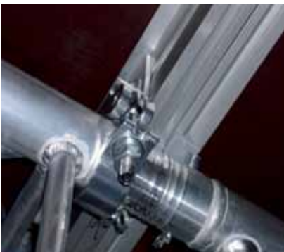
Platform fastening to trusses
