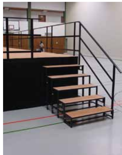
Staircase railings inserted from above
