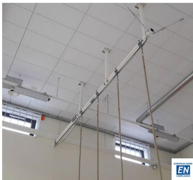
Ceiling suspended construction with rail for hanging climbing ropes. Made of steel profiles, in accordance to DIN 7911-2:1998-12. Protected against corrosion by powder-coating. Standard color of the structure: white.
