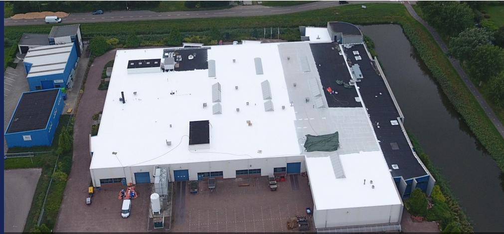
The white Enduris coating reflects solar rays, which resulted in a 3–5% better yield for solar panels positioned on the roof.
